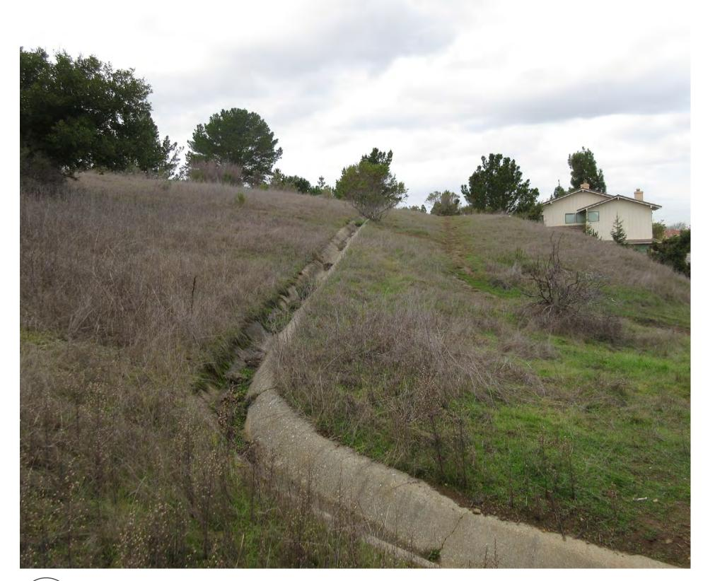
(10) CONCRETE DRAINAGE CHANNEL
